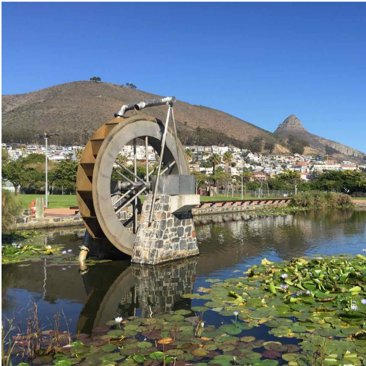
Reconstruction of groundwater fed municipal water infrastructure, now providing environmental and aesthetic benefits. Cape Town, South Africa.
