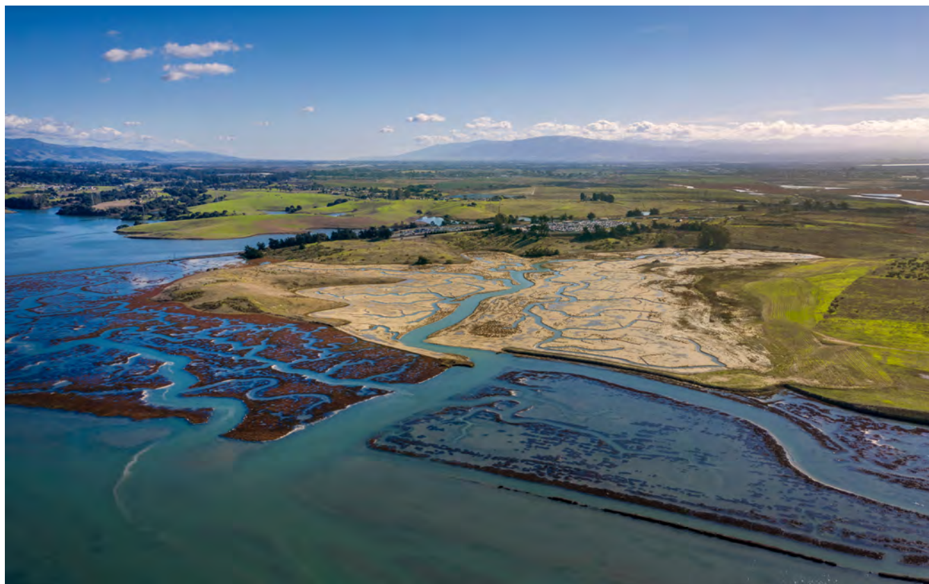
Elkhorn Slough tidal marsh restoration project, U.K., which aims to restore 147 acres of vegetated tidal salt marsh, and native grasslands. Source: Shutterstock.
