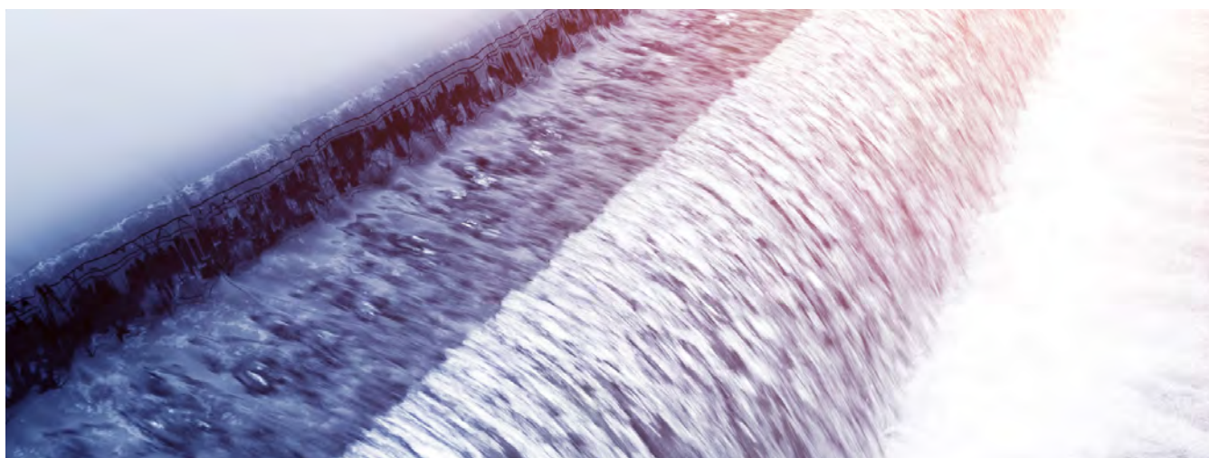
Modern urban wastewater treatment plant. Source: Shutterstock.
