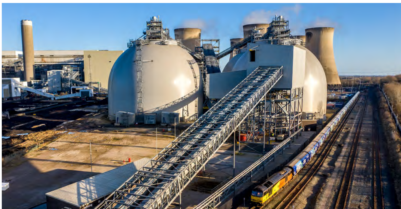
Train delivering fuel to the biomass plant at Drax power station, UK, which is currently investing in BECCS infrastructure. Source: Shutterstock.
