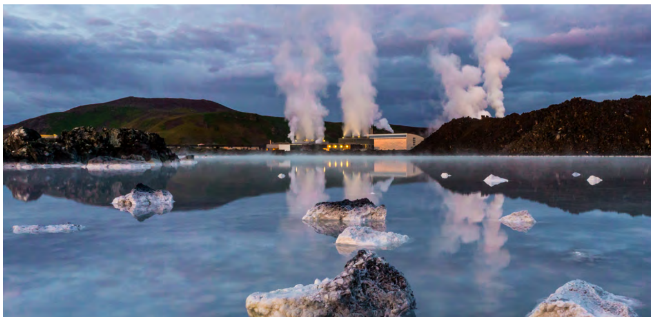
Svartsengi geothermal power plant in Iceland. Source: Shutterstock.
