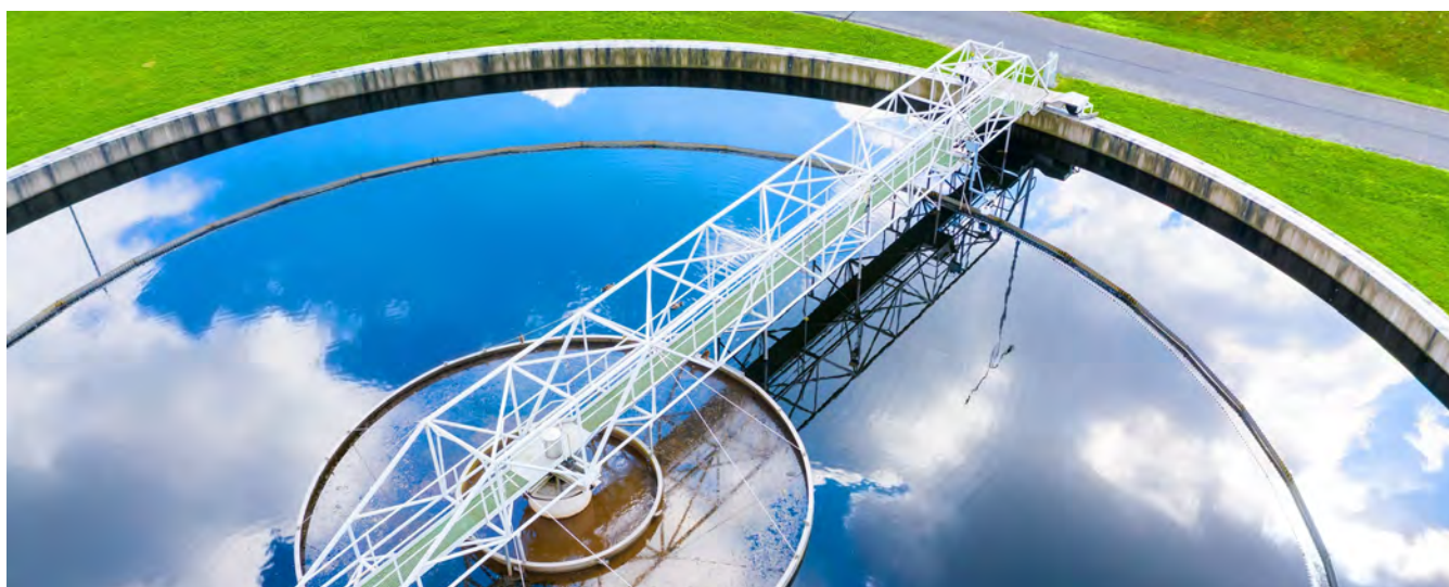
Wastewater treatment tank. Source: Shutterstock.
