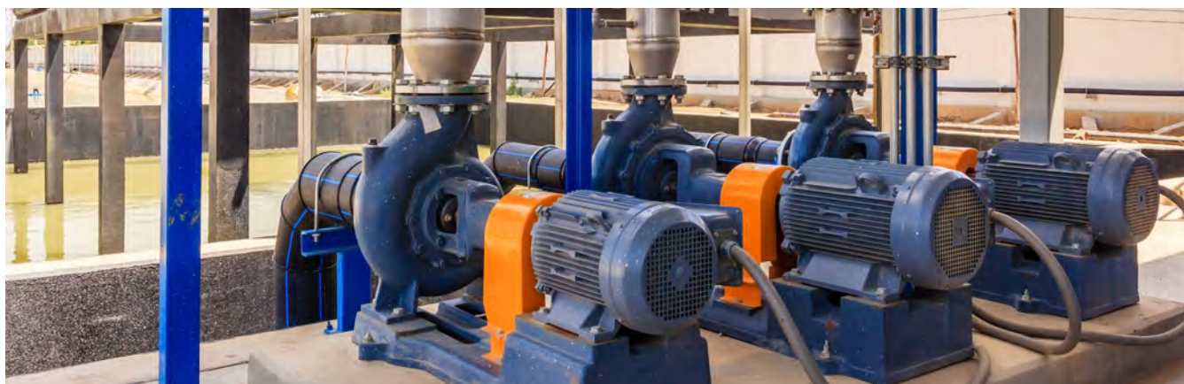
New pumping equipment at an urban wastewater treatment plant can help reduce GHG emissions. Source: Shutterstock.
