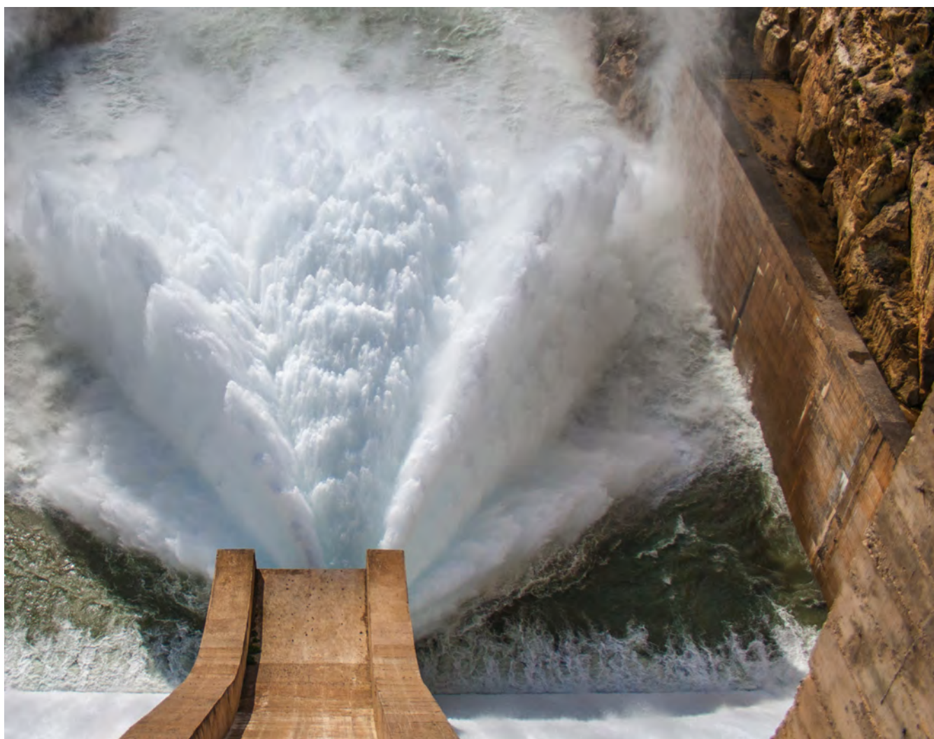
Water being released from a reservoir spillway gate. Source: Shutterstock.
