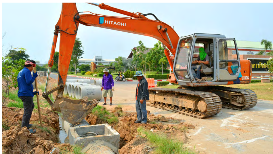
Upgrading the sewer drainage system in Mahasarakham, Thailand. Source: Shutterstock.
