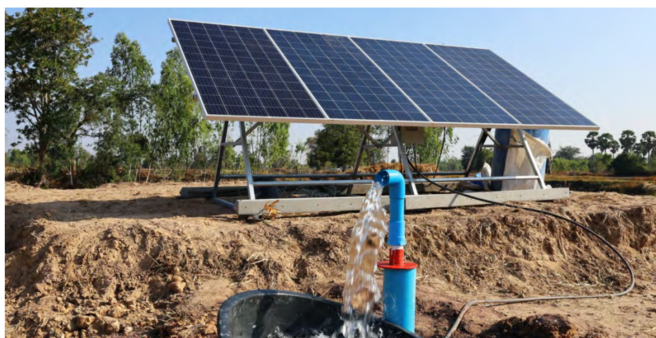
Solar-powered water pump. Source: Shutterstock
