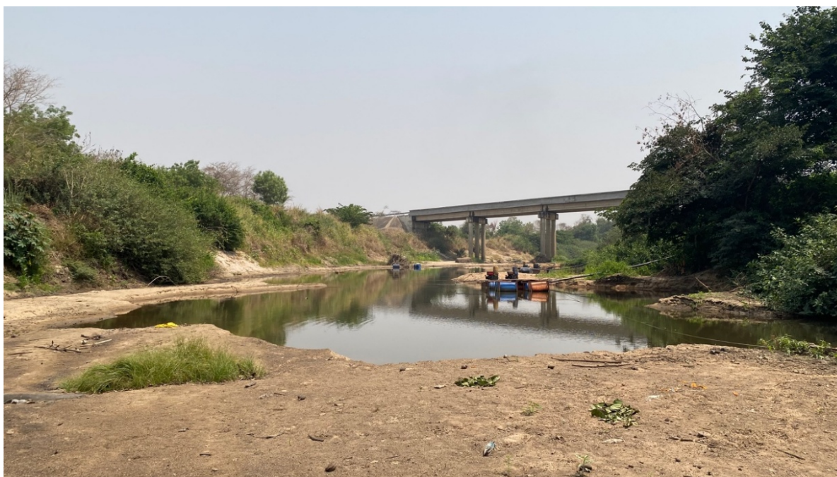
Figure 6: Siltation removal pump on the minor Ogou riverbed implemented by the government. Photo: SIWI.
